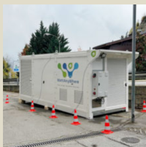
Project WattAnyWhere: generation of clean electricity from ethanol
